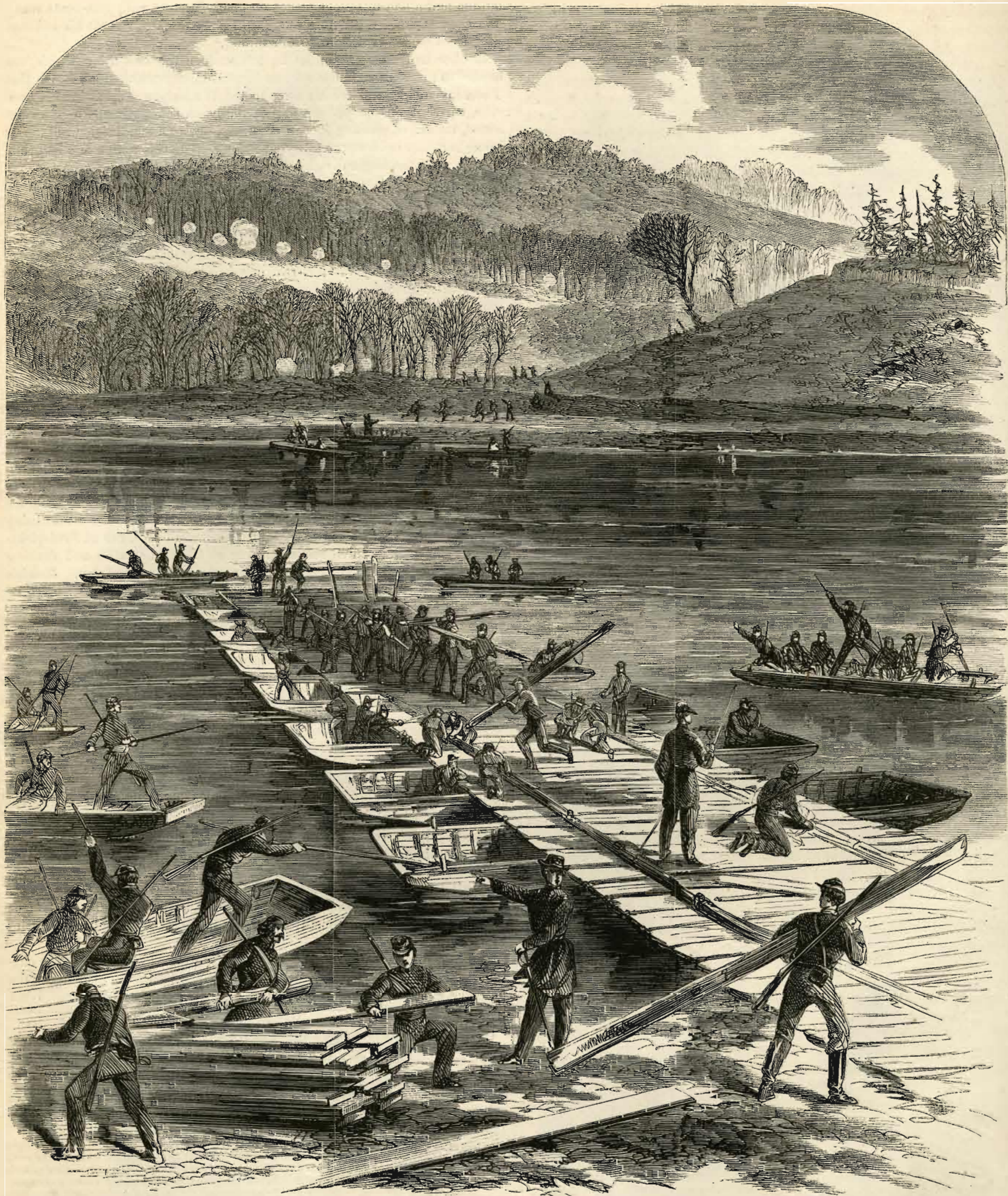
LAYING THE PONTOONS FOR SEDGWICK'S CORPS.
